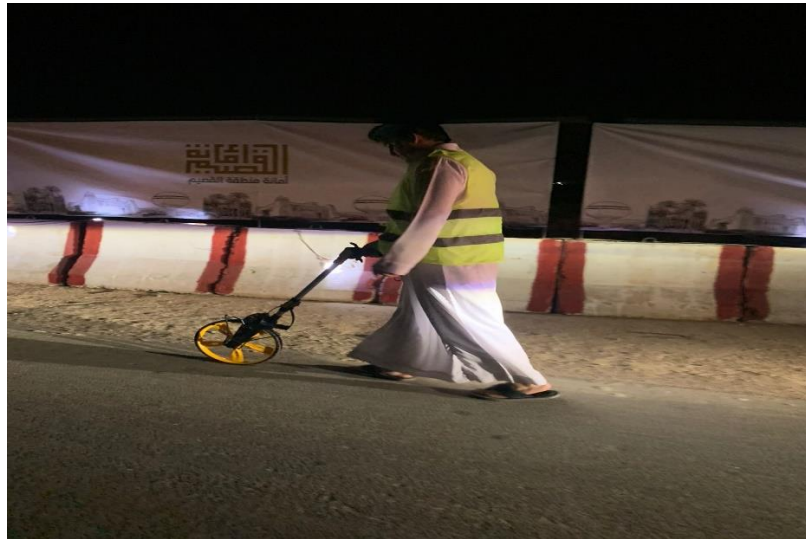
Figure (5): Measuring work zone length using a measuring wheel
