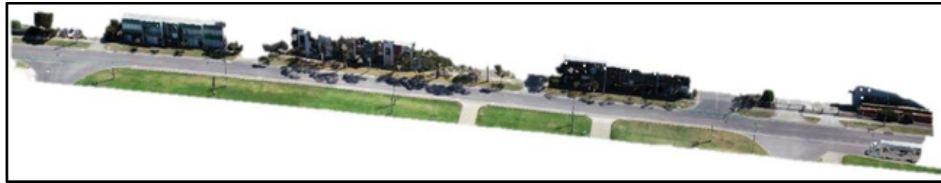
Figure 2: Turner Street reality model developed through photogrammetry.
