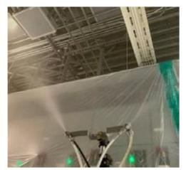
Fig 8. Sealing inaccessible areas behind conduits
