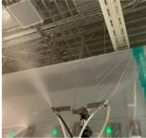
Fig 8. Sealing inaccessible areas behind conduits
