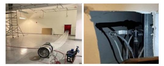
Fig 5. Pressurizing exterior wall
