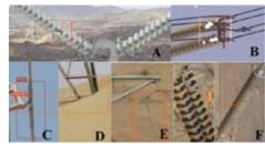
igure 1 A sample of common defects: (A) missing plate along the nsulator chain; (B) Corona discharge (C) damaged strand of the ductor and broken clamp; (D) sand accumulates around tower foo foundation; (E) cable joints, which are more frequently hot spot sensitive; (F) a string of insulators, polluted.
