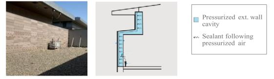
Fig 4. Exterior wall of Mechanical Room
