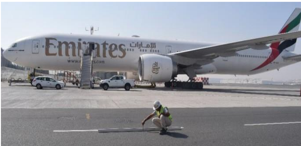
Photo 3: PCI Evaluation of the GSE roads.
