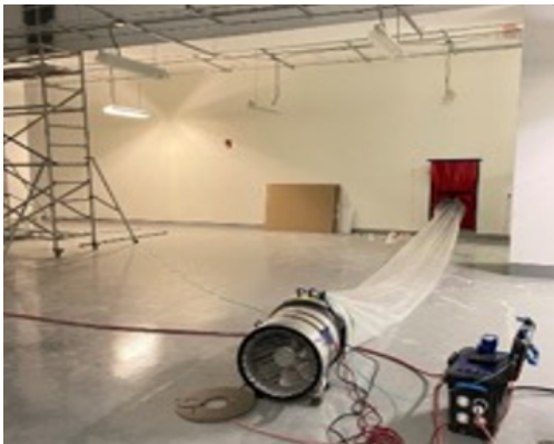
Fig 5. Pressurizing exterior wall
