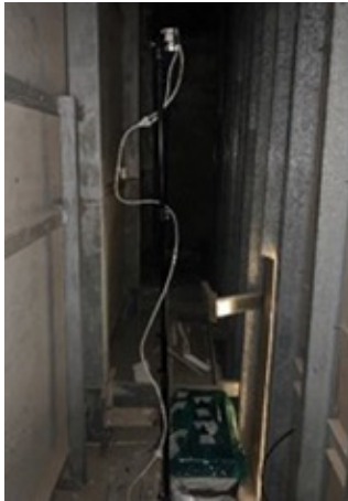
Fig 7. Sealing station inside Exterior Wall
