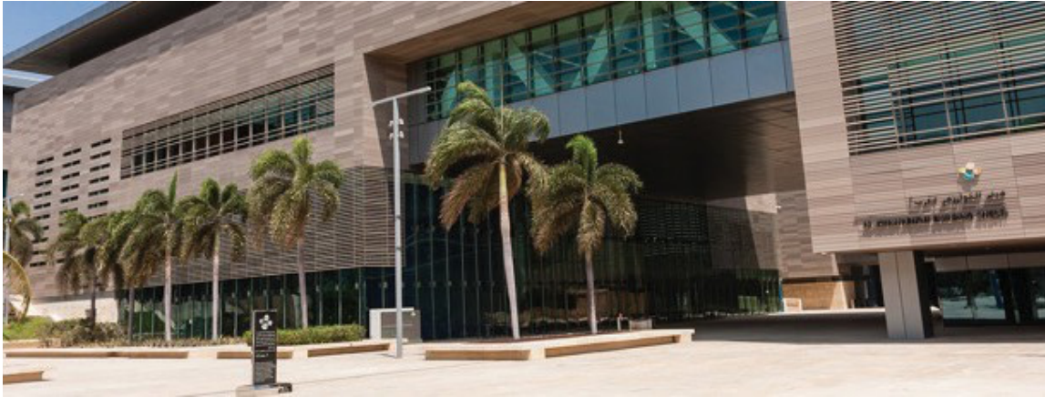
Fig 1. Al Khawarizmi Building at KAUST
