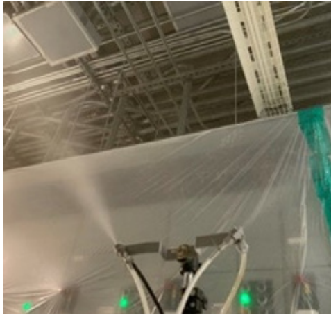
Fig 8. Sealing inaccessible areas behind conduits
