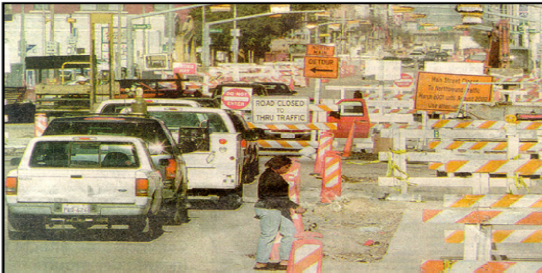
Figure1: Traditional open-cut Trenches construction: Disturbance for Pedestrians, traffic, business and environment [8]
