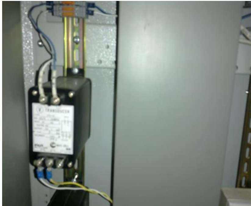
Figure..8: Modified Transducer with 0-1mA is under Testing at the Substation at Najran.
